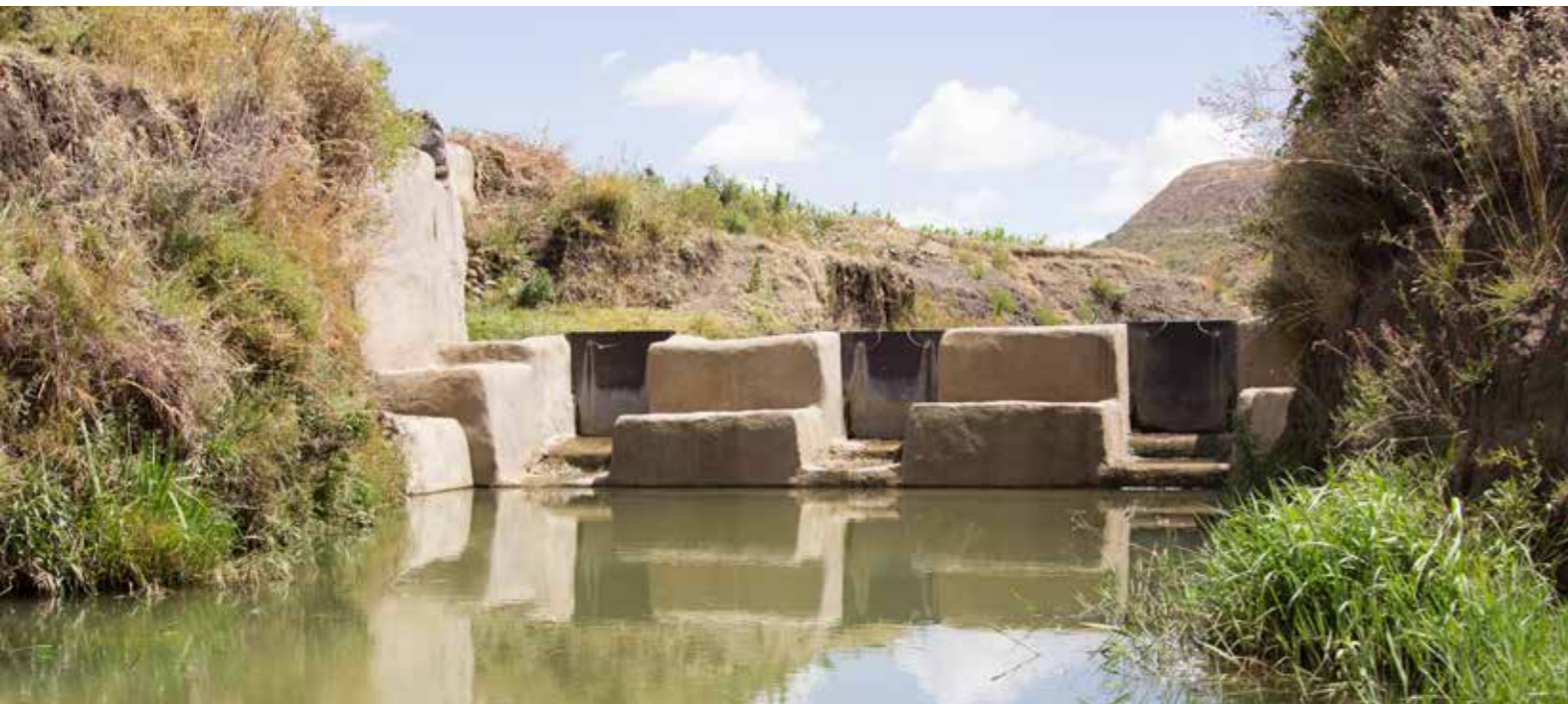
A check dam constructed in Tigray region in Norwegian Church Aid's climate resilience program. Together with various water harvesting schemes the project has proved to increase productivity in agriculture which has again improved livelihoods. The program is part of the national programme that has contributed to Tigray being greener than it has been in 145 years. The Tigray region has won several rewards, the latest being a U.N.-backed award for the world's best policy to combat desertification and improve fertility of drylands. Photo: Hilina Abebe, Norwegian Church Aid Ethiopia
