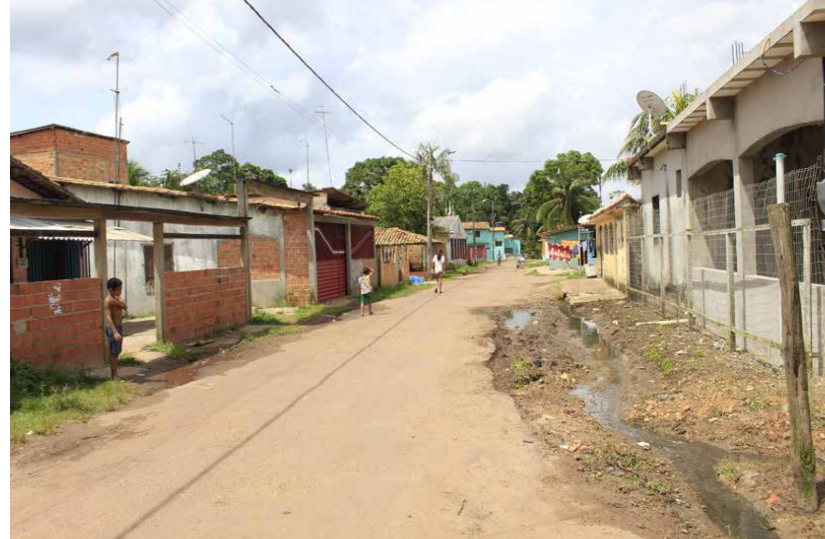
The sanitary situation in Barcarena is very poor. Open pipes lead sewage straight into the road, potentially contaminating clean water reservoirs and spreading diseases. Photo: Daltro Paiva (IEB)
